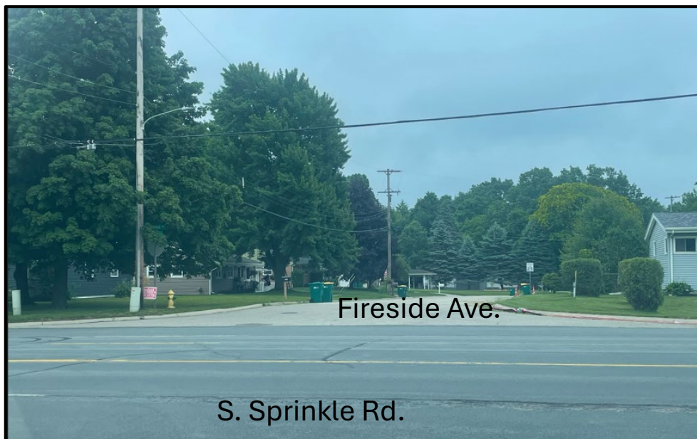
Figure 2: Looking east at entrance to Fireside Avenue from S. Sprinkle Road.
