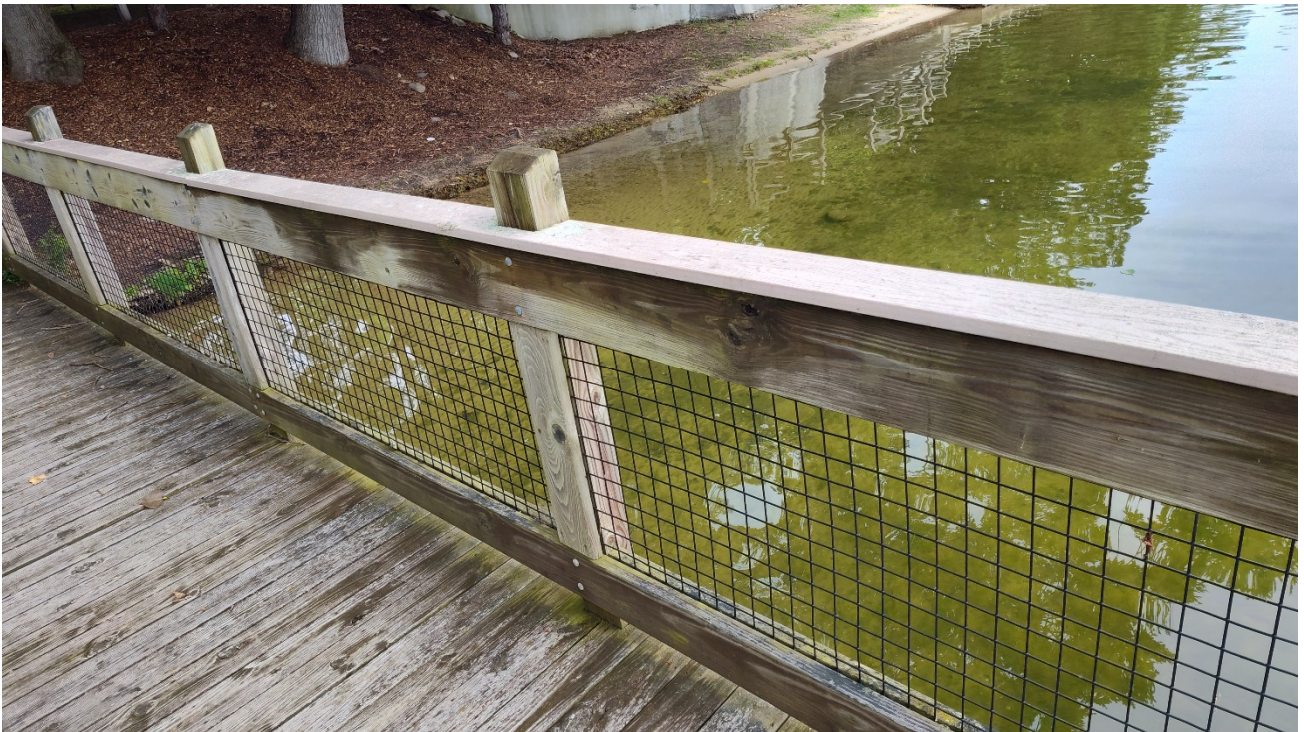
Typical walkway railing
