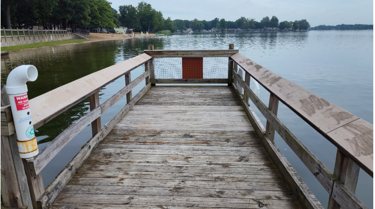
View on pier looking north
