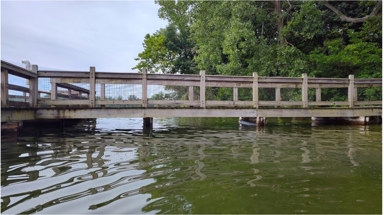
Elevation view of pier walkway looking south
