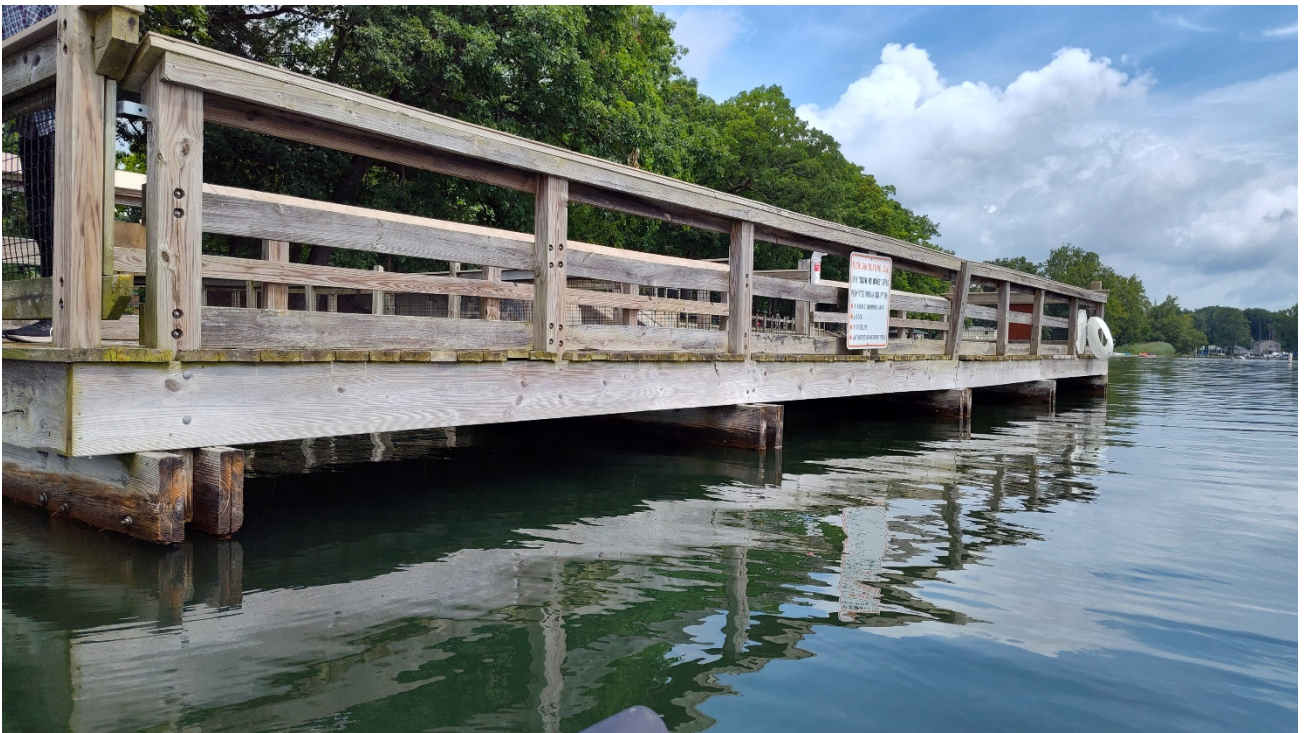
Elevation view of pier end looking north
