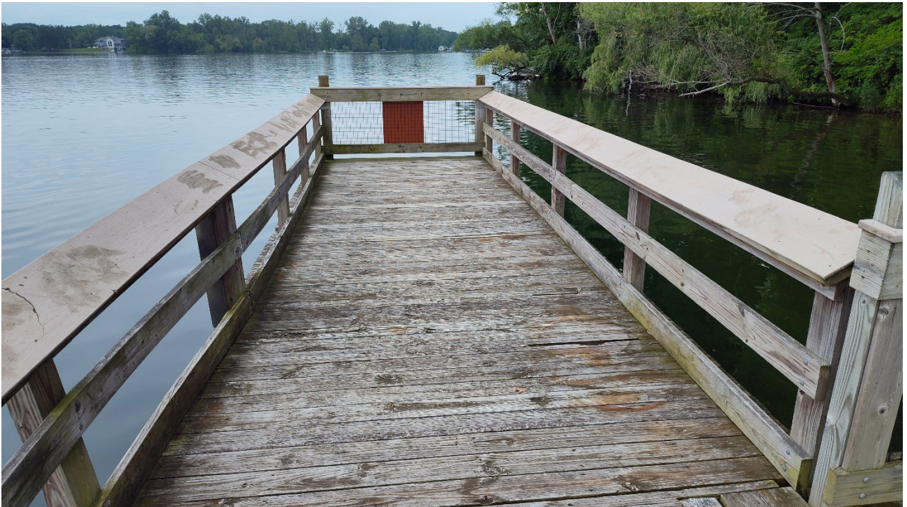
View on pier looking south
