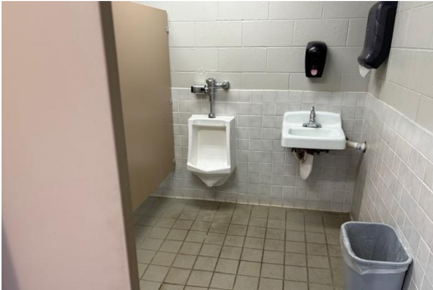
Men's urinal view at door entrance, undersized turn radius, significant signs of wear. Urinal located right next to sink.
