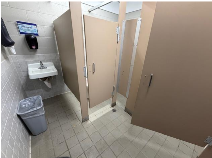
Women's stalls, undersized turn radius and space, open doors interfere with users
