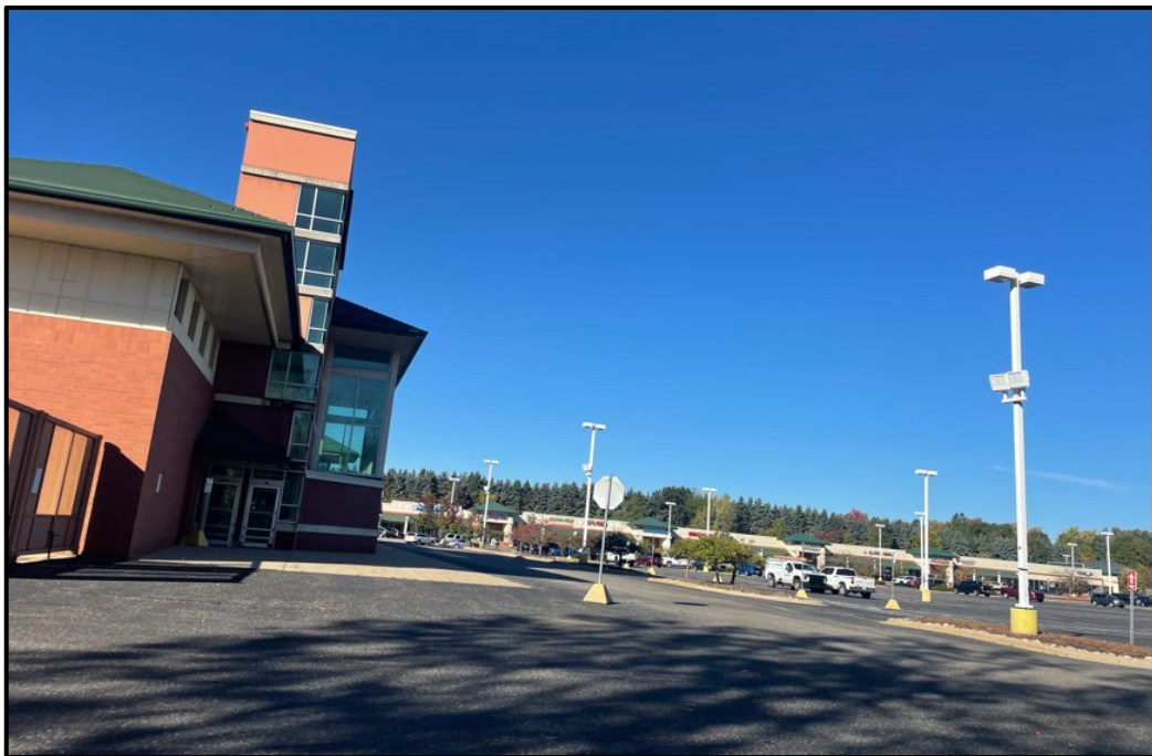
Figure 2. Looking west at façade subject tenant. Parking areas in foreground and background are generally shared within the overall Shoppes at Romence Village.
