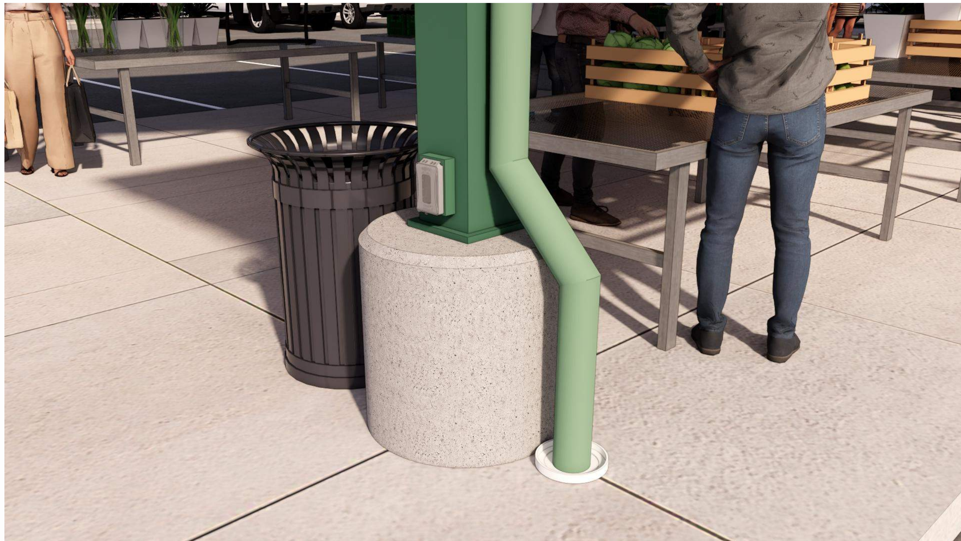
PAVILION PEDESTAL BASE AND ROOF DOWNSPOUT
