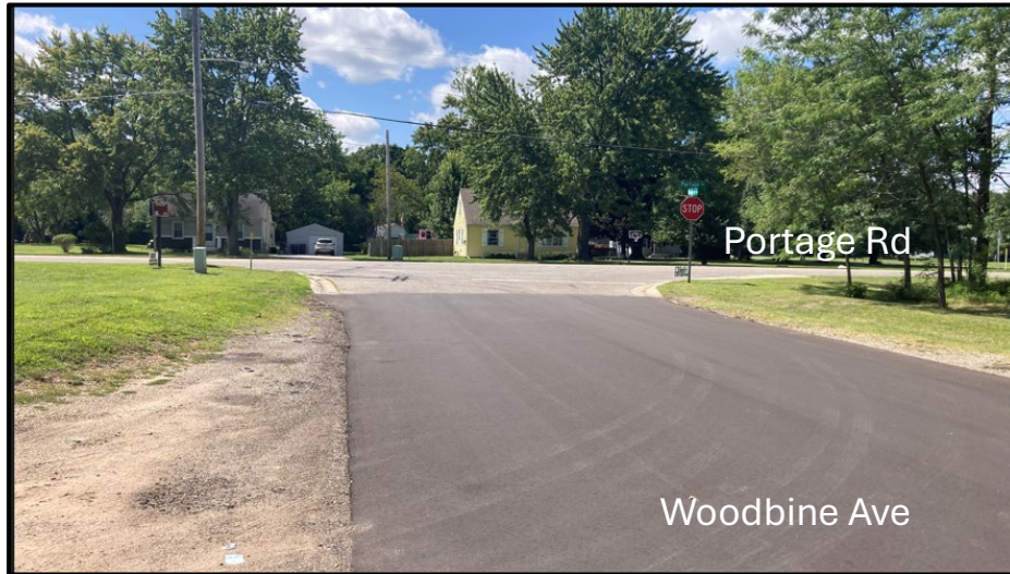
Figure 1. Looking west toward Portage Rd & Woodbine Ave. intersection.
