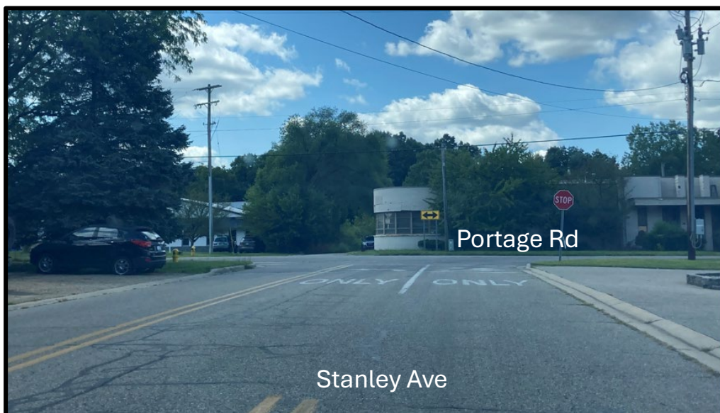
Figure 6. Looking west toward intersection of Portage Rd & Stanley Ave.
