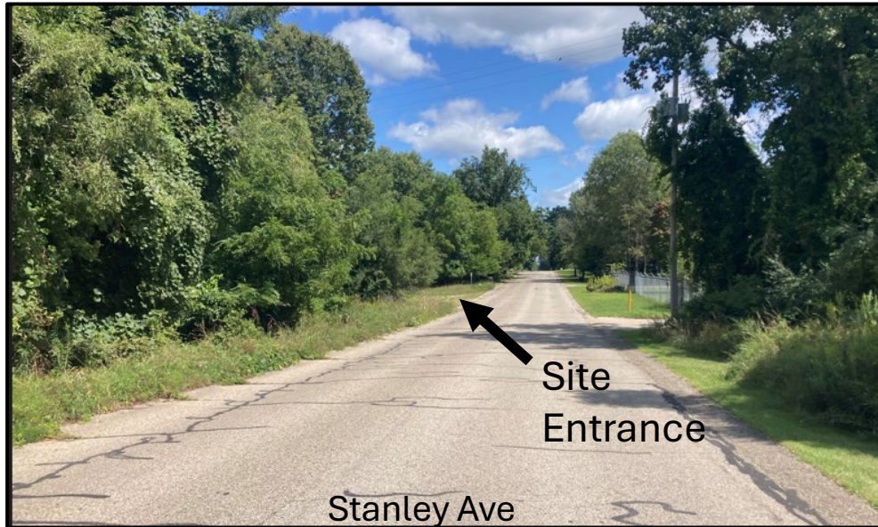
Figure 7. Looking east along Stanley Ave. toward second site entrance.
