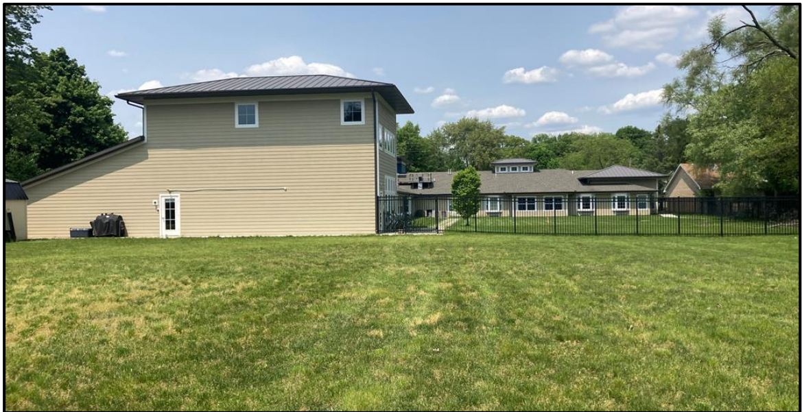
Figure 6. Looking north at the back elevation of the Beacon Point building and lawn space. Proposed development building addition will add onto the most foreground building wall.
