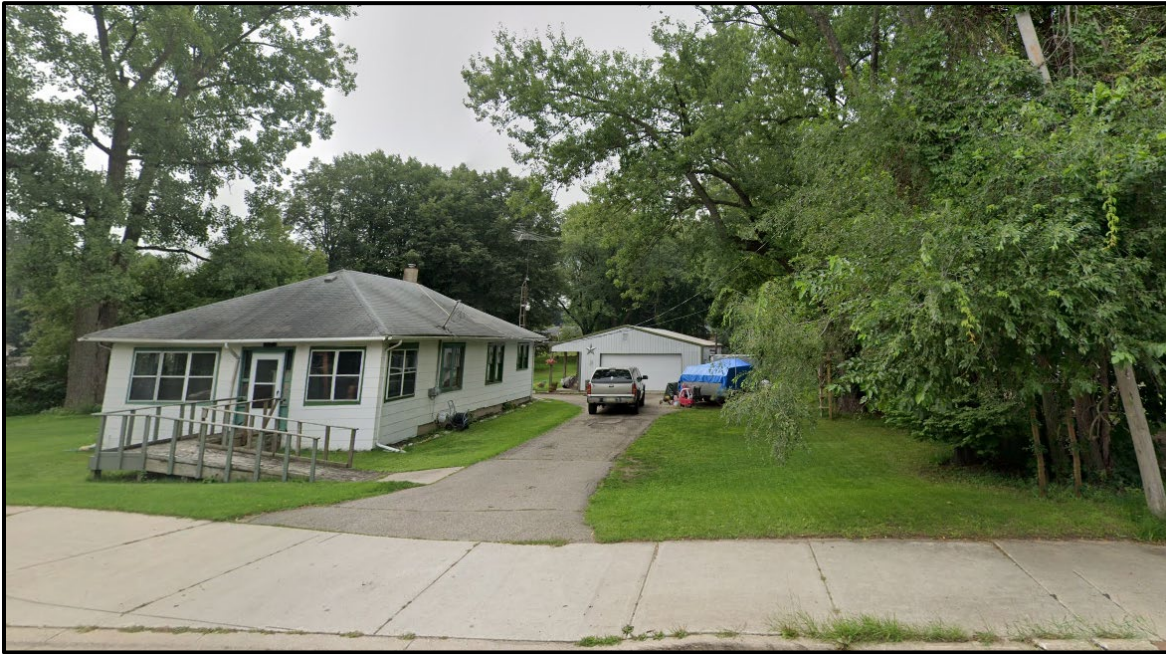
Figure 3. Looking south at subject house and detached garage.
