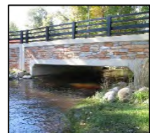
Figure 4: Three-sided Box Bridge
