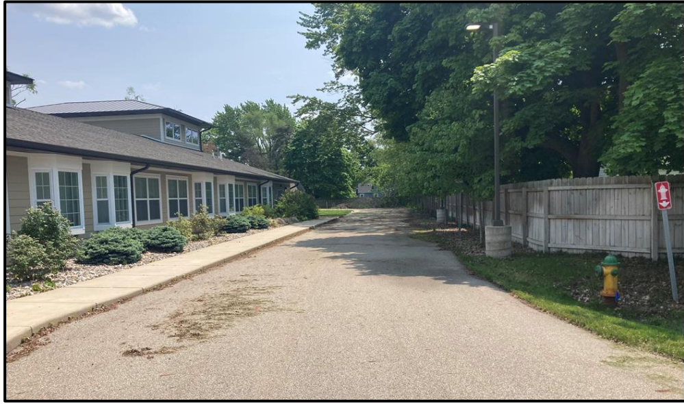
Figure 7. Looking south along the service drive of the Beacon Point site. The service drive will be reused in its existing location. The existing six-foot tall (approx.) wood fence in this picture is planned to be increased to eight feet in height.
