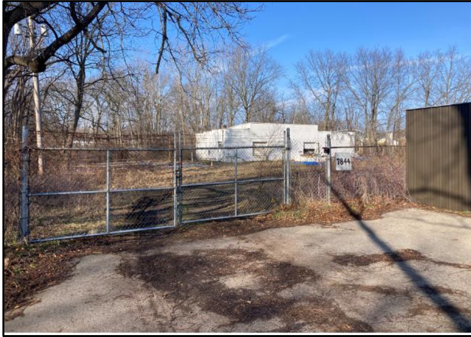
Figure 3. Looking northwest at subject property behind fence gate. Building (background) in picture behind fence is located within site. Covered parking (in front of fence) for Fire Station is located to the right.
