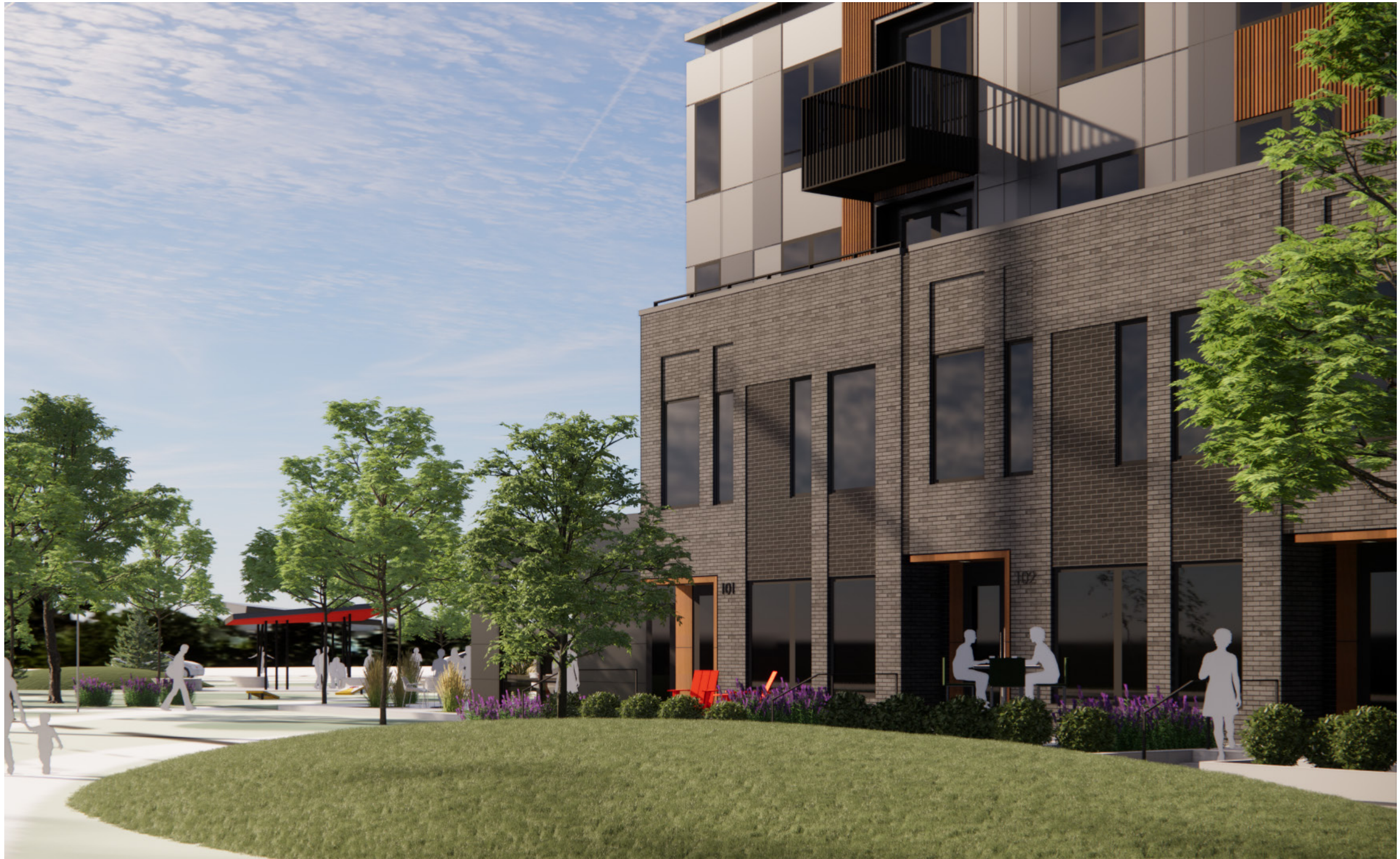
SOUTH WALKING PATH AT BUILDING B
