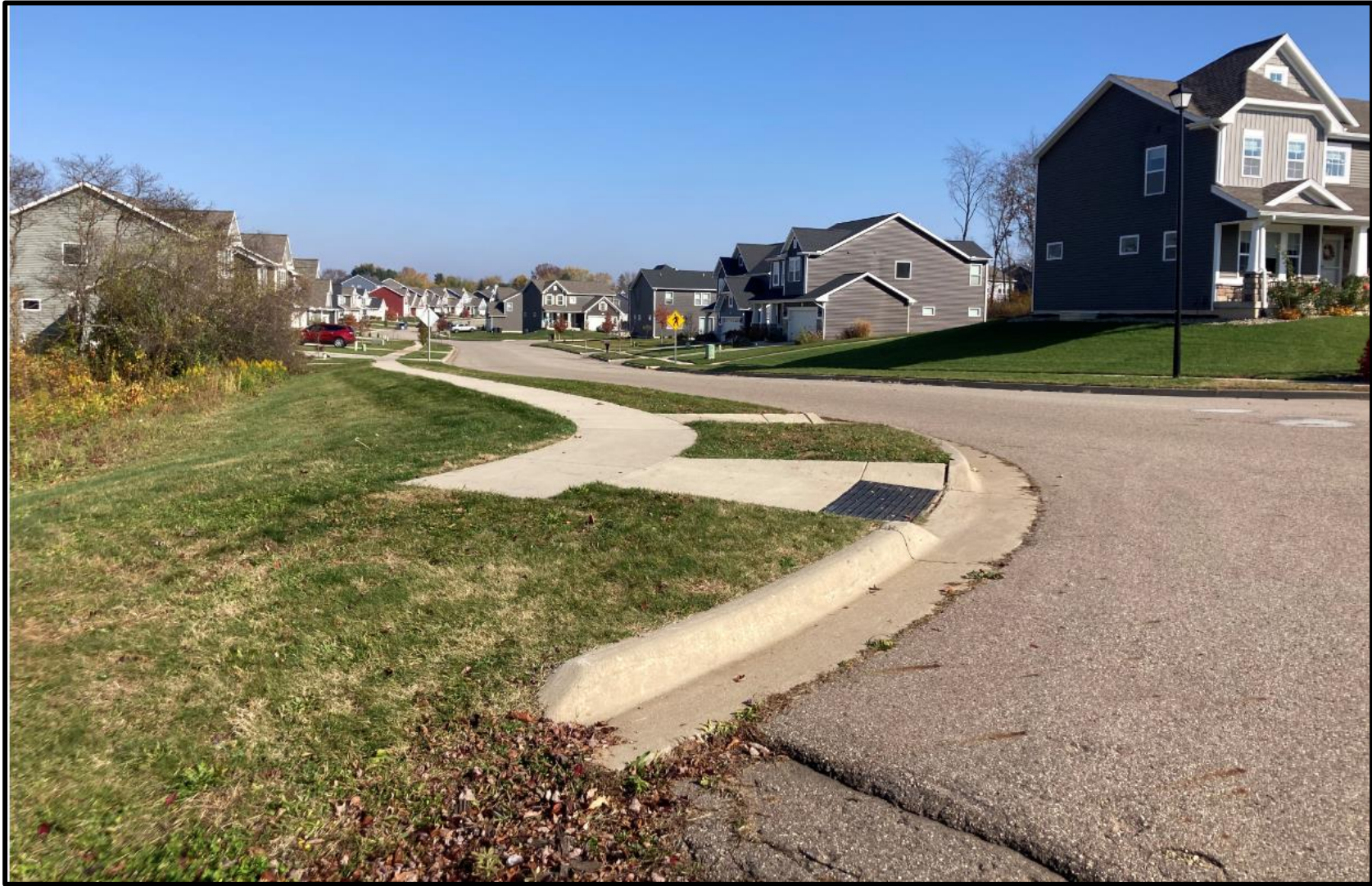
Figure 4. Looking east along Copperleaf Trails at homes within Phases 1, 2 & 3. Foreground street curb-cut will be extended with new street (Landrum Trail).
