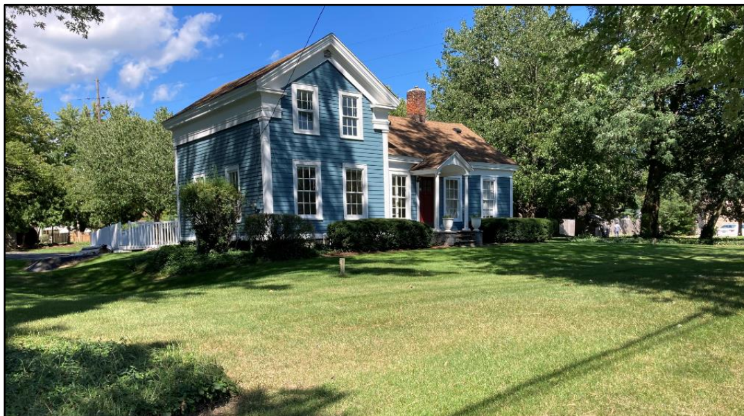
Figure 3: Façade elevation of 515 E. Centre Avenue. Built in 1853, listed on the City of Portage Historic District.
