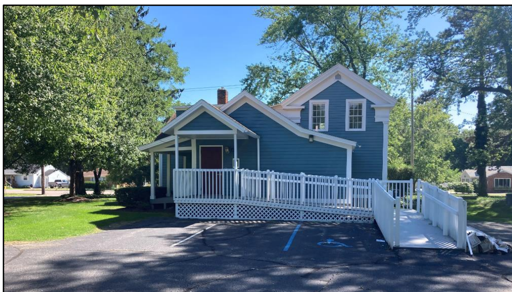
Figure 4: Rear elevation of 515 E. Centre Avenue. Kingston Drive to the left (East).
