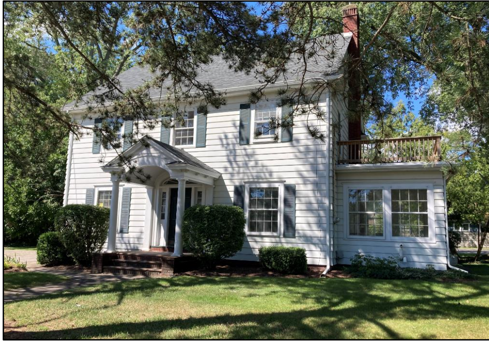
Figure 1: Façade elevation of 505 E. Centre Avenue. Built in 1927.
