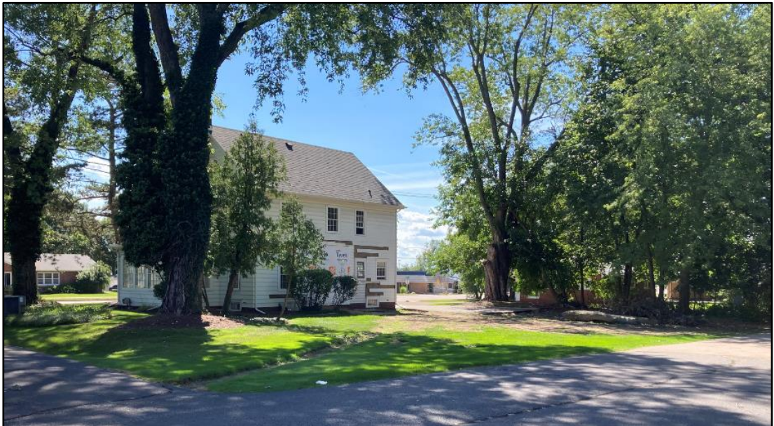
Figure 2: Rear elevation of 505 E. Centre Avenue. Private, common parking lot to the right (north).
