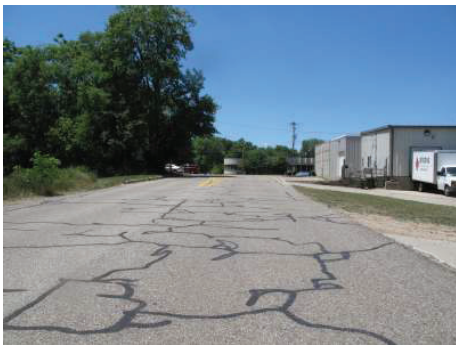
Stanley Ave. - Looking West
