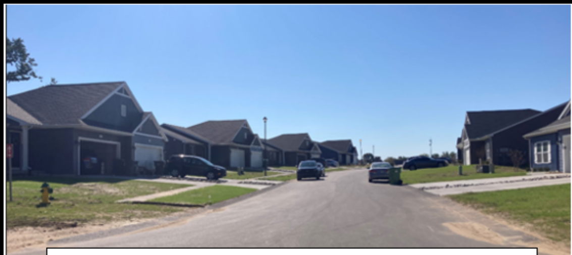
Phase 1 (Attached Units). Units 1-22, Attached homes; Duplex Buildings. (Facing South)
