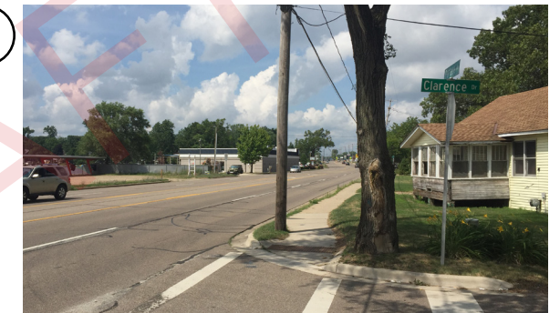
Where sidewalks exist, they are substandard width, forced to negotiate with existing elements like trees, utility poles, and buildings for extremely limited space.
