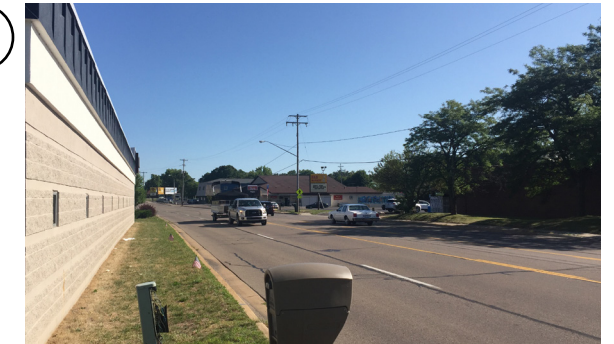
A major pinch-point exists at the Cove restaurant where, due to the expansion of Portage Road over the years, only 8 feet of space is left between the curb and the building.
