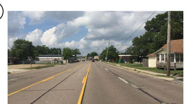
The absence of crosswalks in the isthmus area, across five lanes of high-speed traffic, presents a difficult environment for pedestrians and cyclists to cross.
