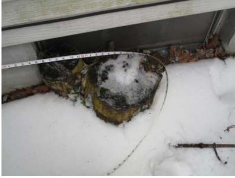
Tree Stump by Foundation
