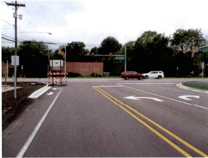
Zylman Avenue - Looking West - Traffic Signal
