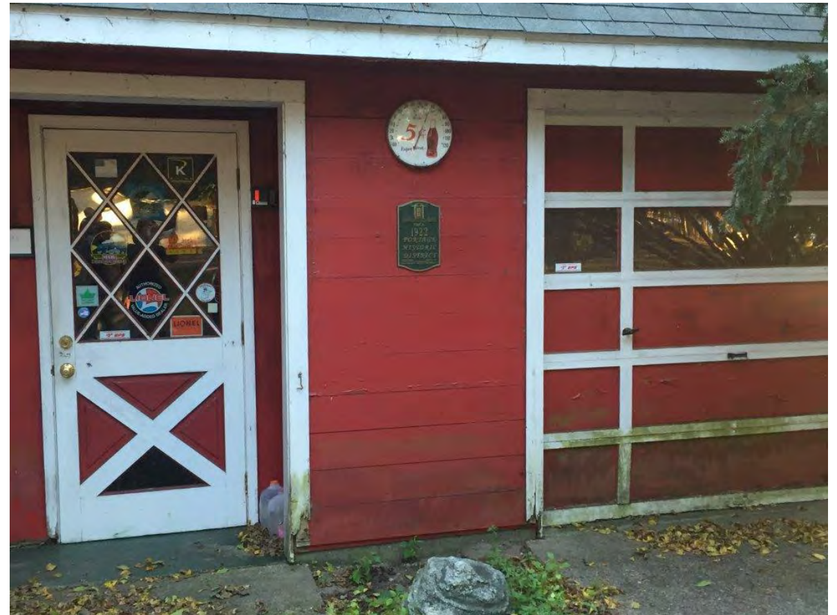
North Entrance to Train Barn on Remainder Parcel
