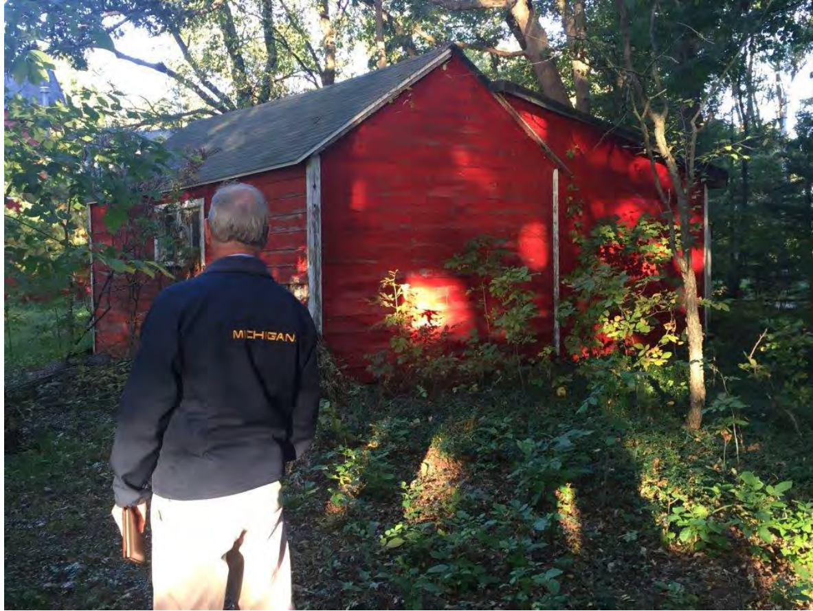
South side of Granary
