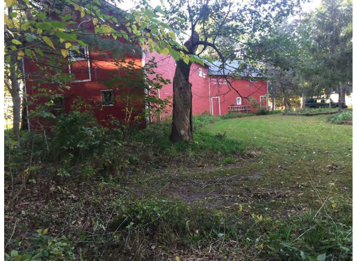
Train Barn from Street View – North - West
