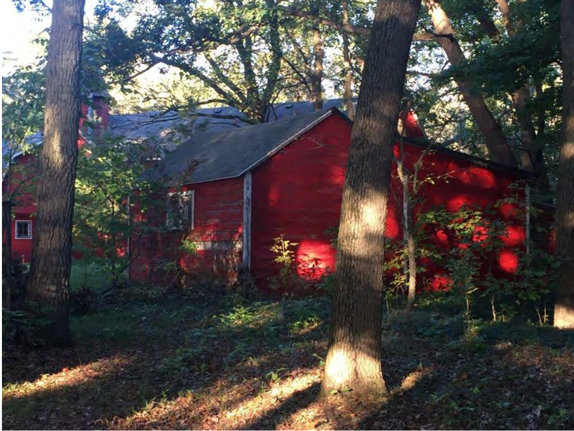
South side of Granary
