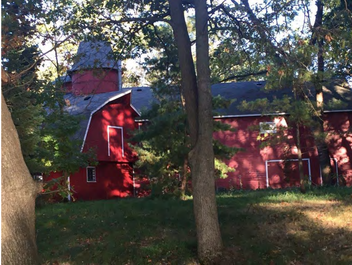
Train Barn on Remainder Parcel View- from lake toward East (West side of Barn)
