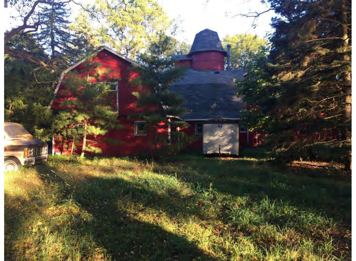
View of Train Barn from lake toward North - East
