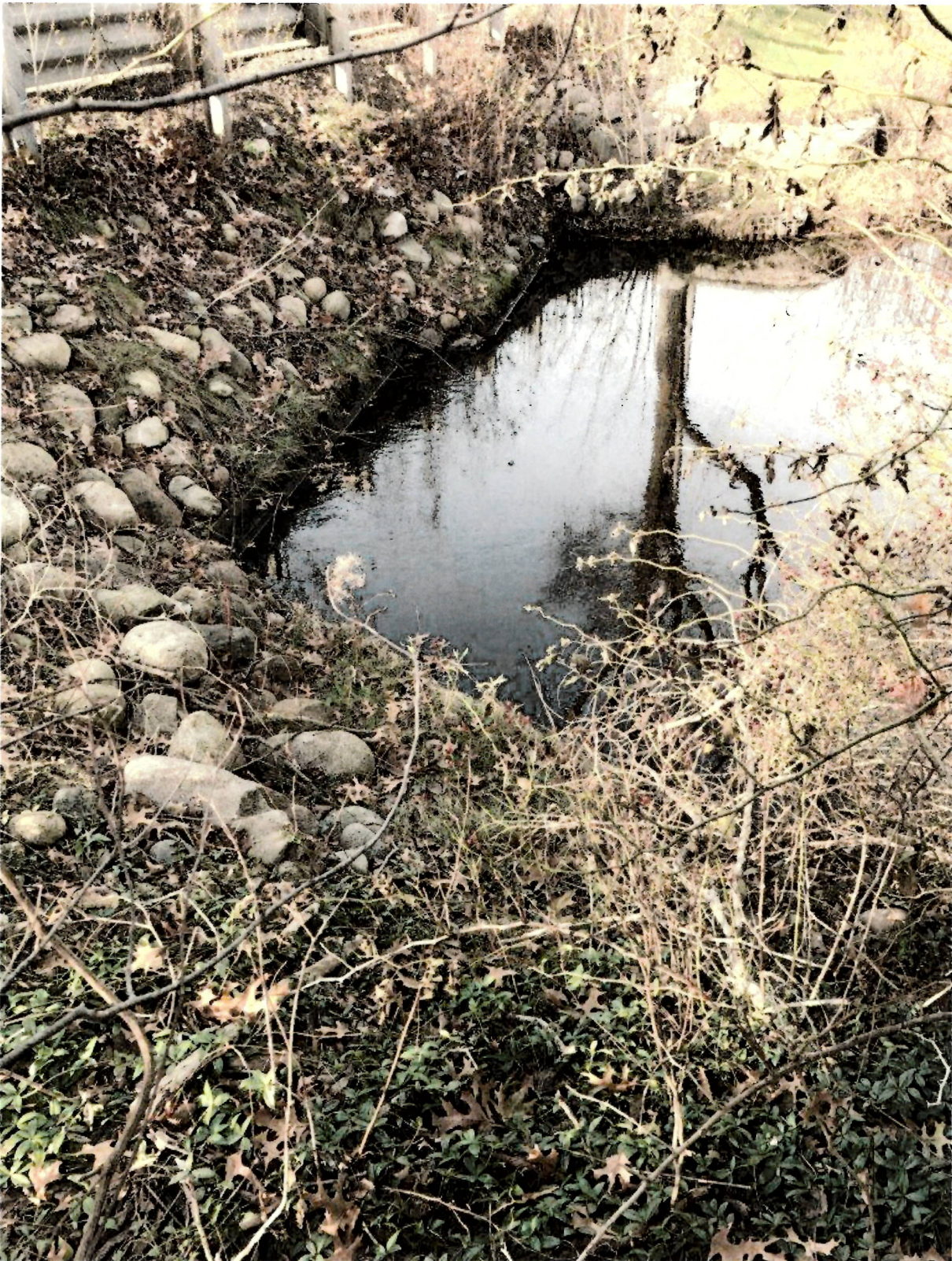
Oakland Drive – West side of culvert
