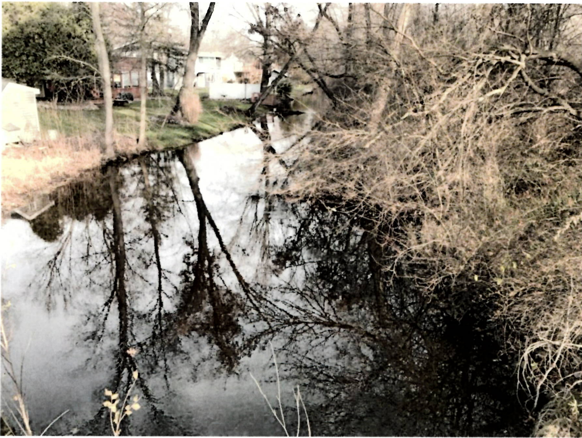
Oakland Drive – East side of culvert, looking downstream
